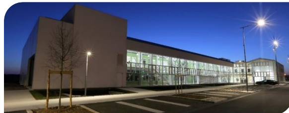
The Tipee building on the Atlantech low-carbon park in Lagord - Photo credits: Frédéric LE LAN / CDA La Rochelle
